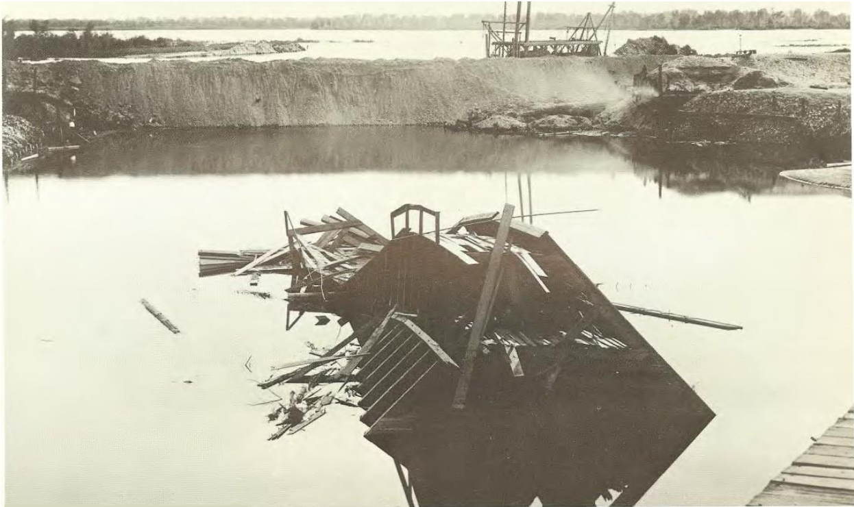
Rock and earth fill barrier was constructed at Imperial Canal inlet after the gates were destroyed in the 1906 flood.
