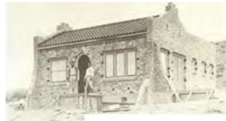
Government housing under construction in Boulder City, 1931.
