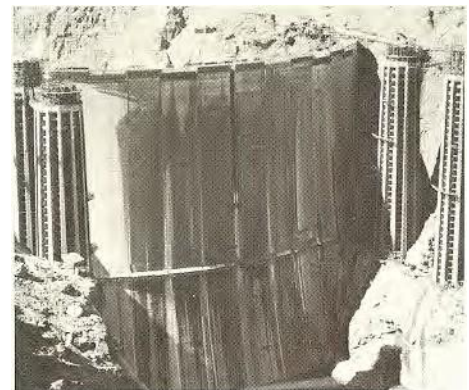
Upstream face of Hoover Dam and intake towers.
