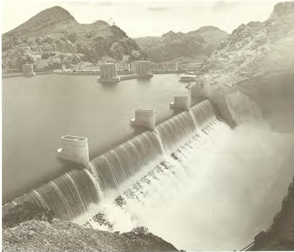
Water rushing over the Nevada spill way at peak capacity of 13,944 cubic feet per second and 4-1/2 feet above spillway gates, July 1983.
