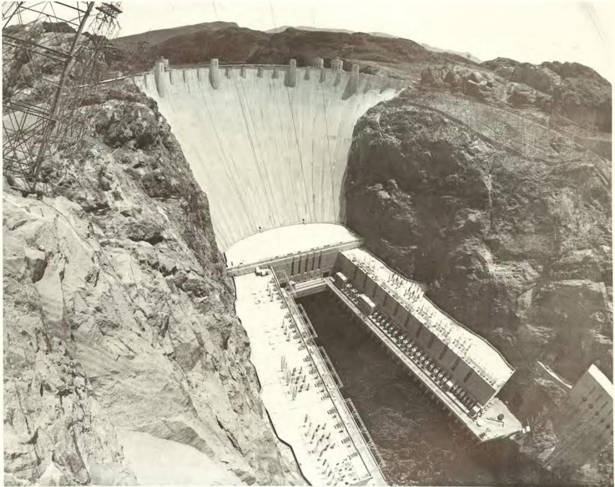
Hoover Dam controls and regulates the Colorado River for multipurpose uses.
