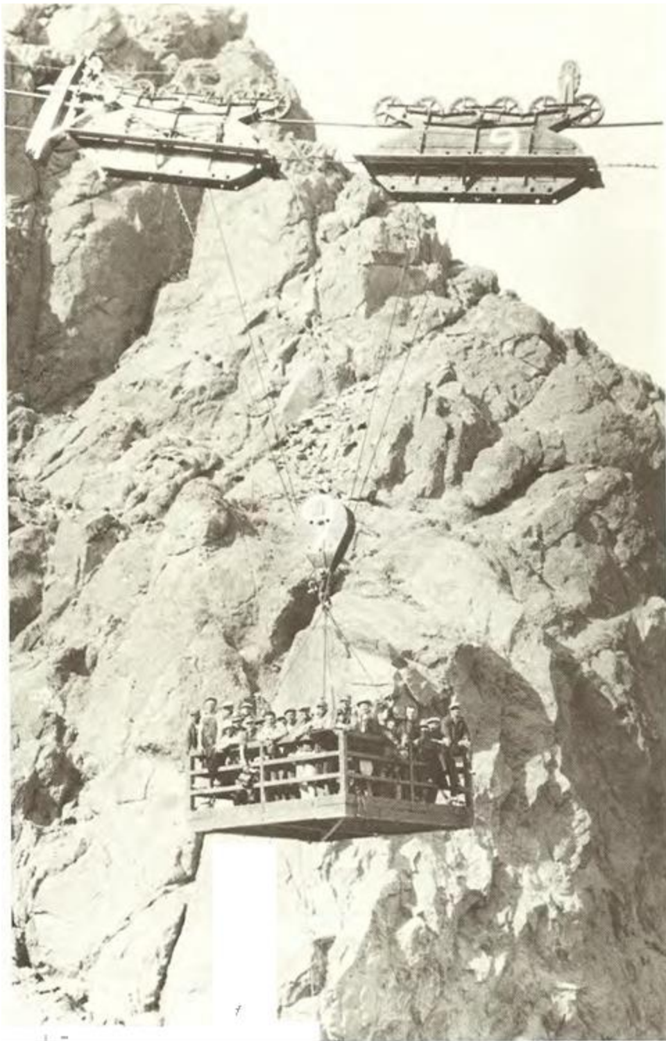
Cableway lowered men and equipment into Black Canyon to work on the dam.
