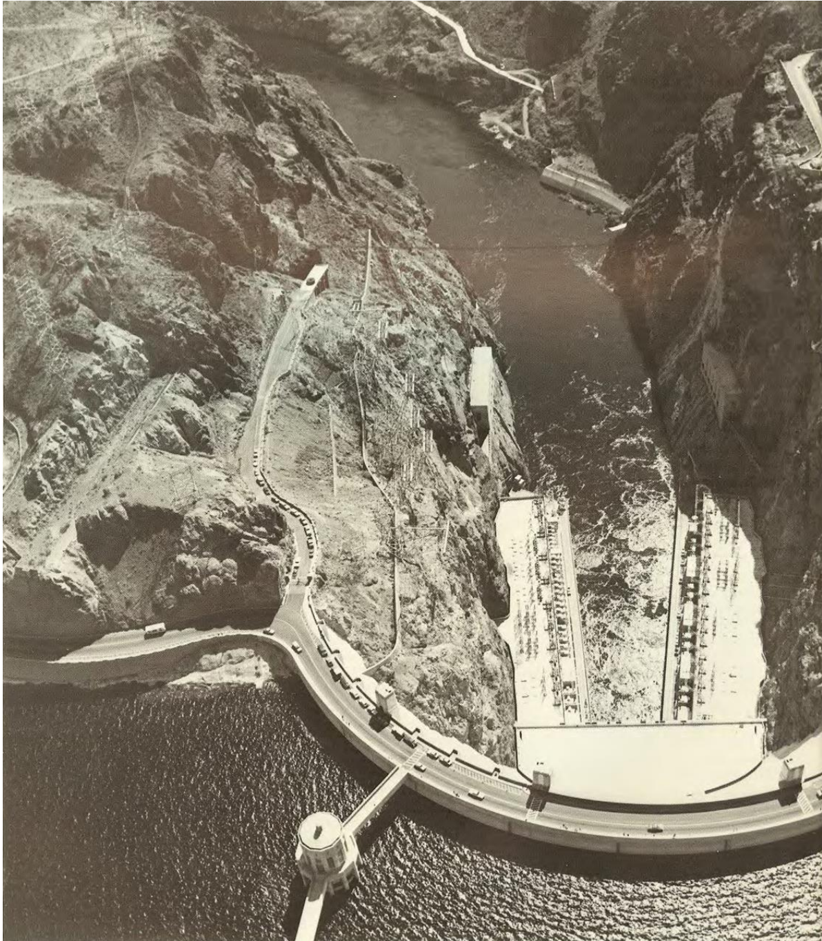
Aerial view of powerplant and Colorado River far below crest of Hoover Dam.
